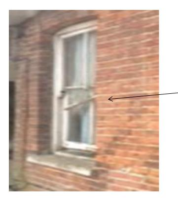
The wood at the bottom of the top sash loose, which meant that the glass was just hanging in the frame with a risk of it falling out
