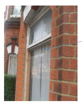
The repair carried out by the occupant was not effective and created an excess cold hazard.
